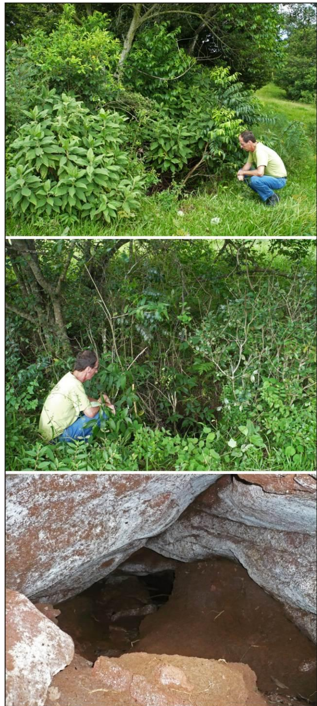
Fig. 11: Big craters of the Cassel property. Top and middle: craters may be 2.0 meters deep. Bottom: more than 4.5 meters deep, in the sound sandstone, half-clogged tunnels with collapse features show off.
